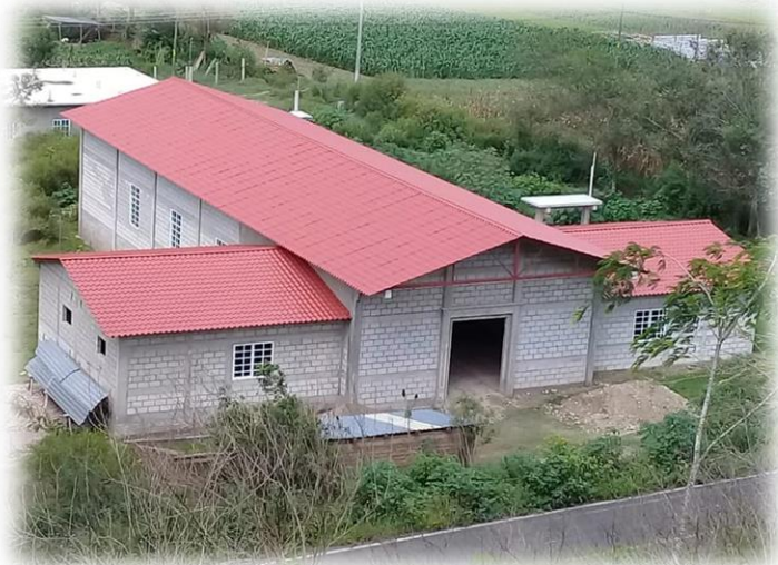
The dental clinic is the right wing in front of the water tank platform
